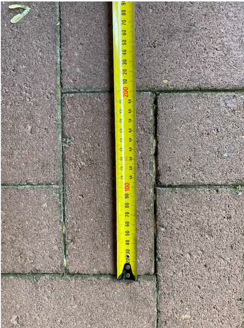
Existing Station Paver 200x100mm
