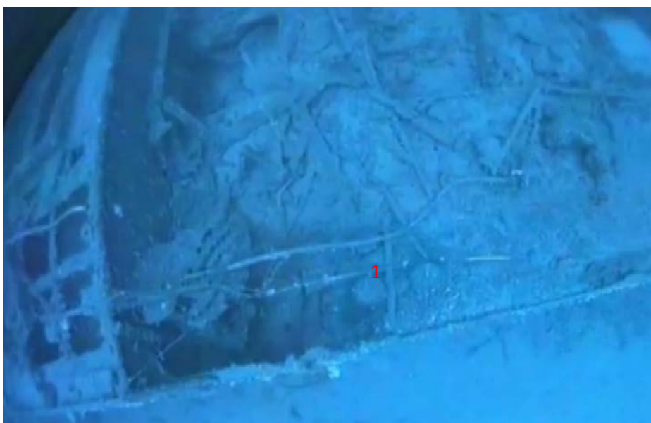
Figure 58: Bitts starboard side and handrails (1) (Image: CSIRO 2023 - 07834)
