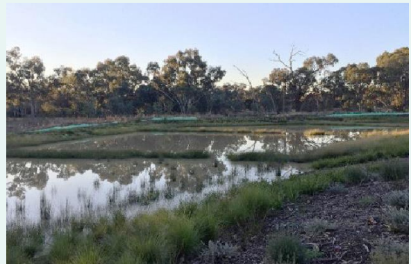
An artificial wetland constructed in a new urban development. Photo: Helen P. Waudby/DPIE
