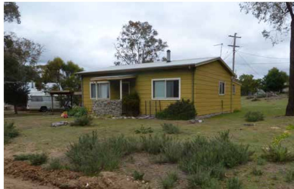
Figure 27 – Existing Cottage 10 (Tract 2016)
