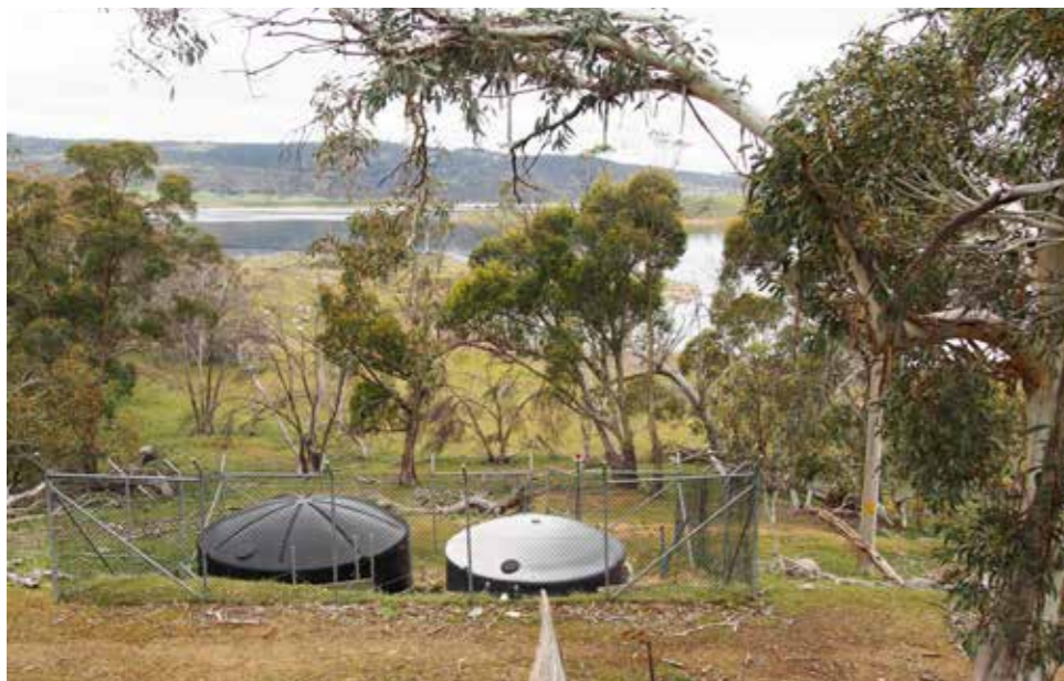
Figure 33 – Existing rainwater tanks (Tract 2016)
