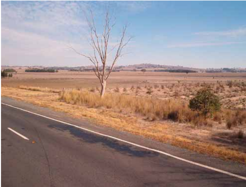
Plate 12: Road restricting surface and shallow groundwater flow causes salinisation on upslope side of road.
