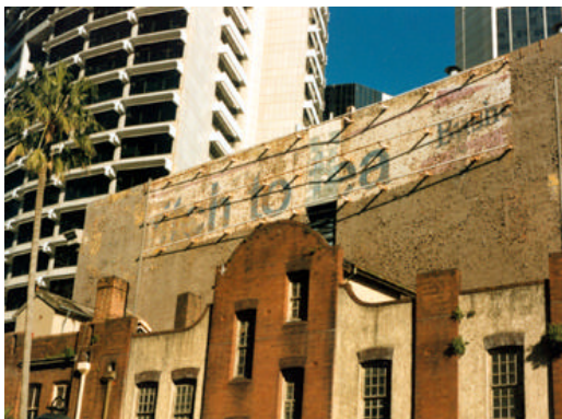
‘Switch to tea’ sign on the northern facade of the Bushells Building before conservation, 1999.
