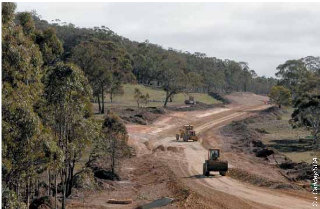
Figure 6.1 Construction of unsealed road showing topsoil stockpiles ready for respreading
