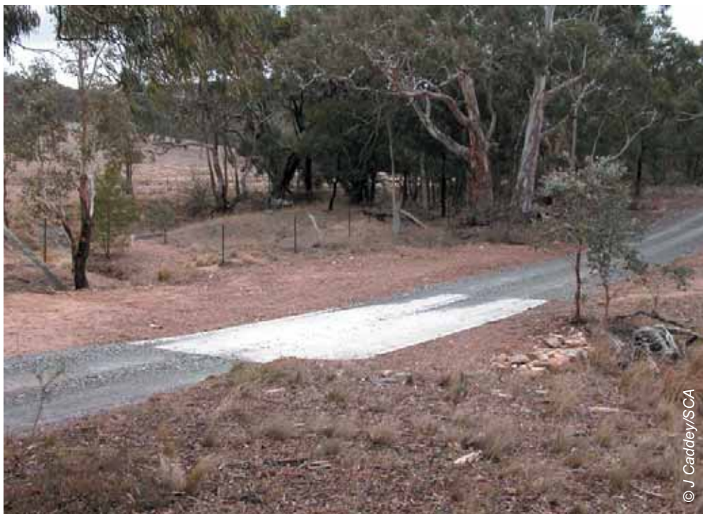
Figure 5.12 A simple causeway across a drainage line
