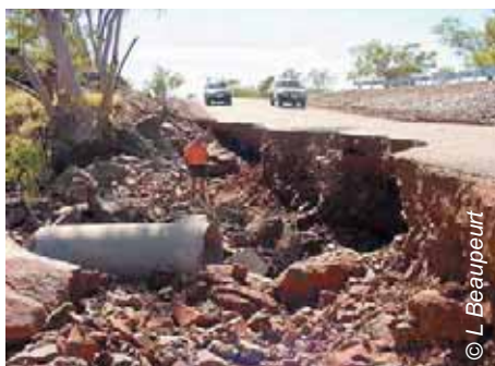
Figure 5.13 The failure of a side track watercourse crossing following a storm event
