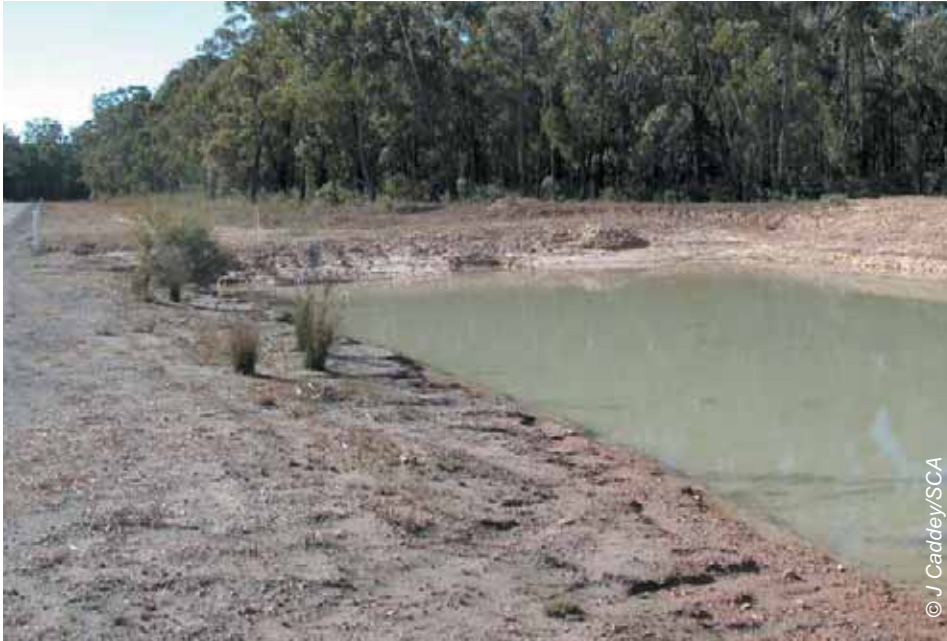
Figure 6.5 Temporary sediment basin adjacent to an unsealed road
