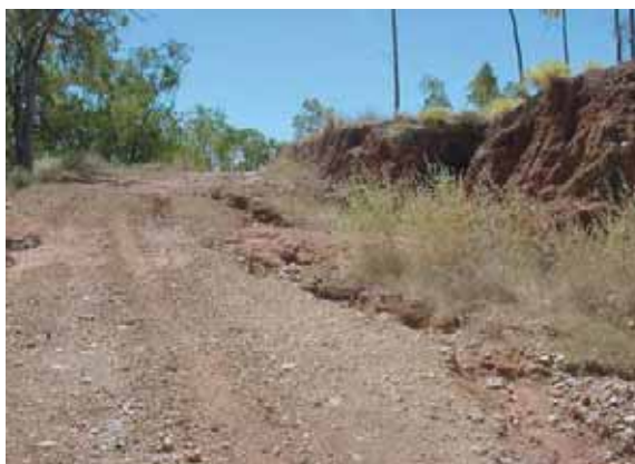
Figure 5.4 The result of a lack of drainage on a quarry access track
