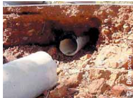
Figure 5.13 The failure of a side track watercourse crossing following a storm event
