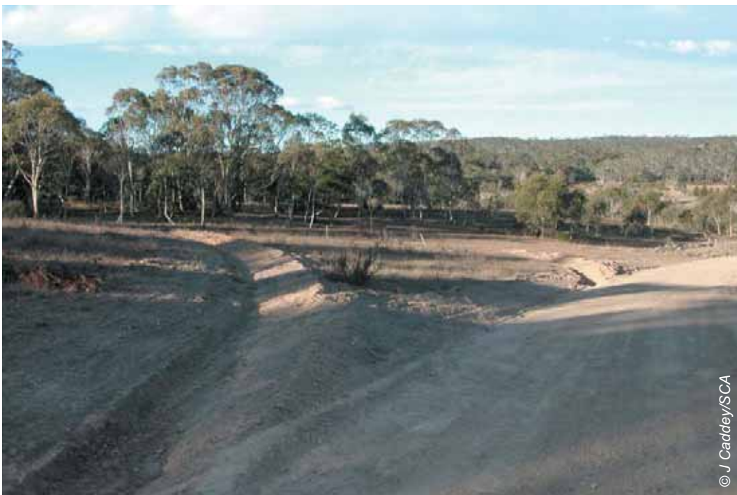
Figure 5.10 Mitre drains
