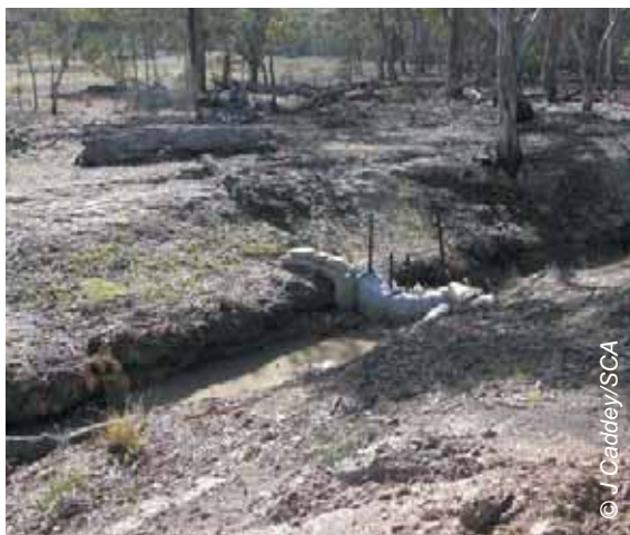
Figure 6.3 Temporary sediment trap
