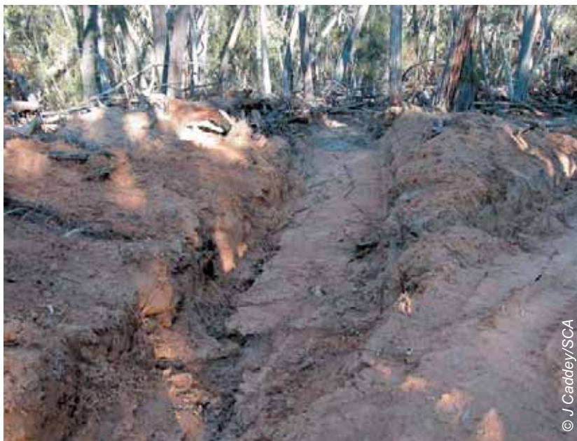
Figure 7.1 Sediment build-up in a mitre drain
