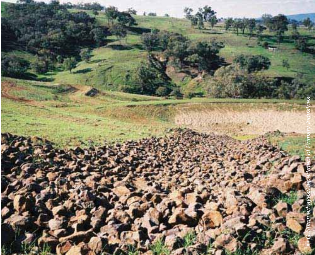
Figure 6.1 Rip-rap rock waterways conveying runoff to a sediment basin
