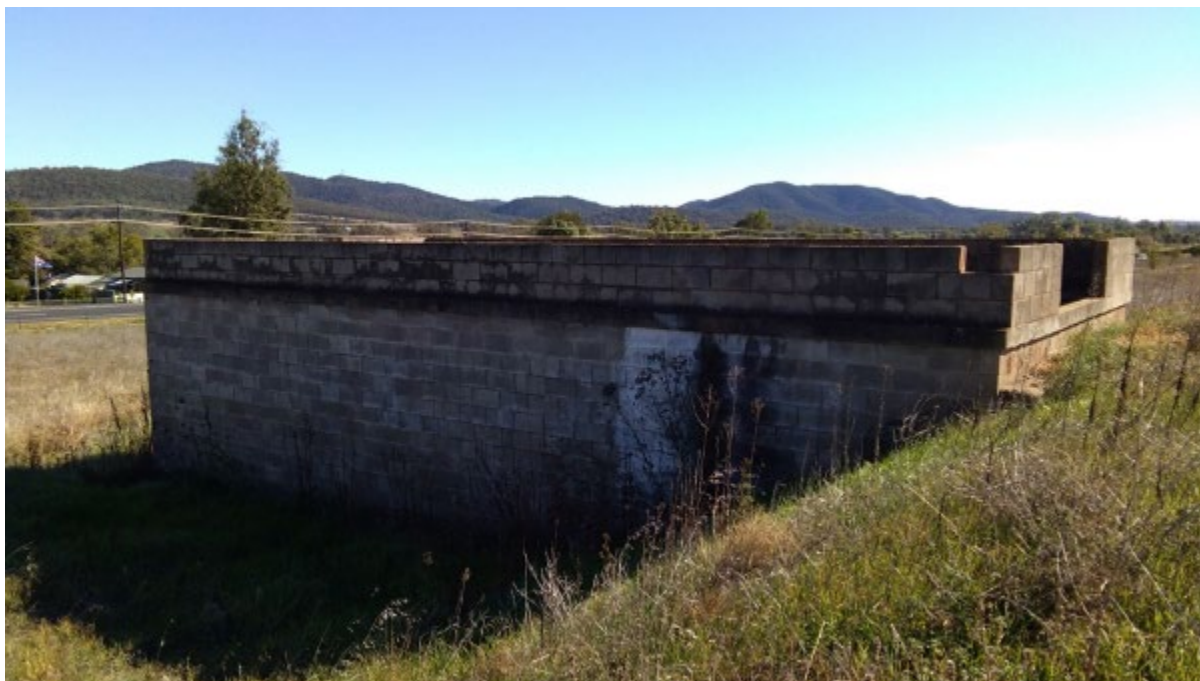
Photo 6 Better block shed and loading ramp from a former chicken farm on Military Barracks Block. M Billington/DPE
