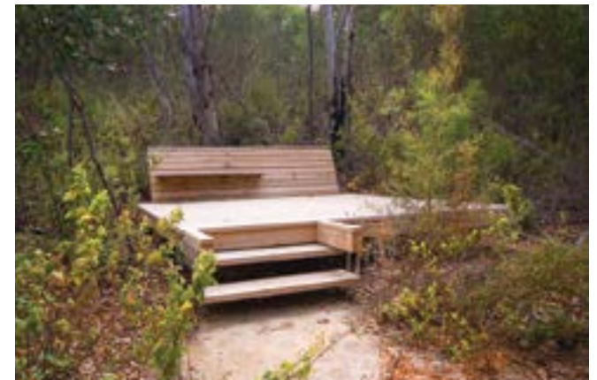
Camp Deck. Photos: Shannon Architects.
