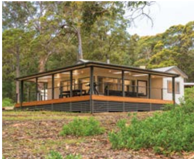
Existing Yellow Rock beach houses. Photos: John Spencer/DPIE.
