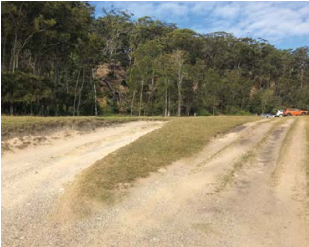
Erosion to Maloneys Beach foreshore due to unauthorised vehicle access. Photo: DPIE.
