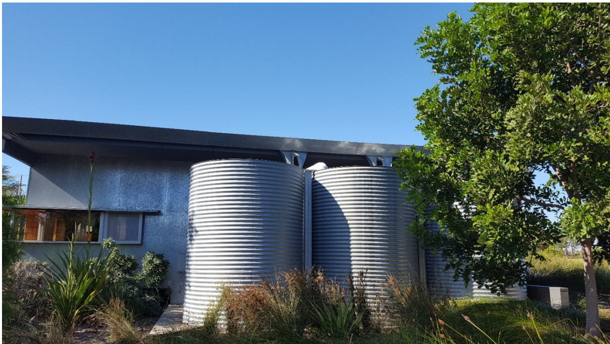
Figure 2 Rainwater tanks at Bungarribee
