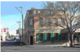
Former Haymarket Hotel prior to restoration, 1995 and following restoration, 2003. Images Ian Wynd and David Rowe.
