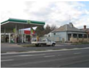
Development of the Victorian cottage as a shop saved it from demolition. Image Sinclair Croft, Bathurst Regional Council
