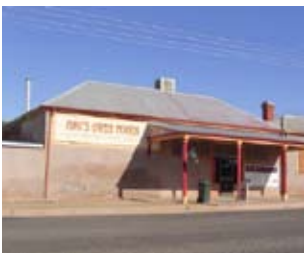
Frontage before and after verandah restoration. McDougall & Vines (2005) 'Broken Hill New South Wales - Verandah Program - 1998 - 2005 Summary Program'
